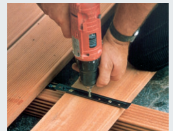
fixing of decking
